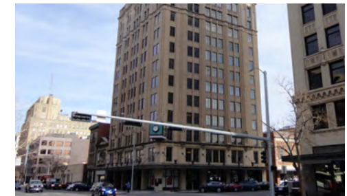
Federal Trust Building 134 S. 13th Street For Lease $14.50/SF MG 492-4,978 SF Marc Hausmann Link to Listing #25341898
