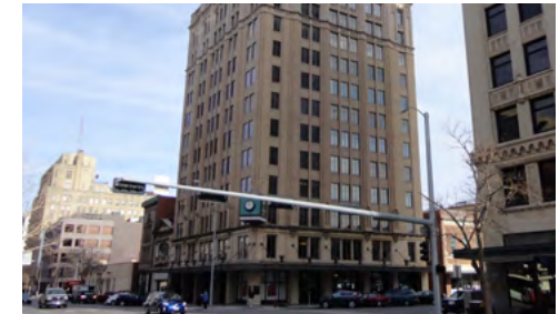
Federal Trust Building 134 S. 13th Street For Lease $14.50/SF MG 492-4,978 SF Marc Hausmann Link to Listing #25341898
